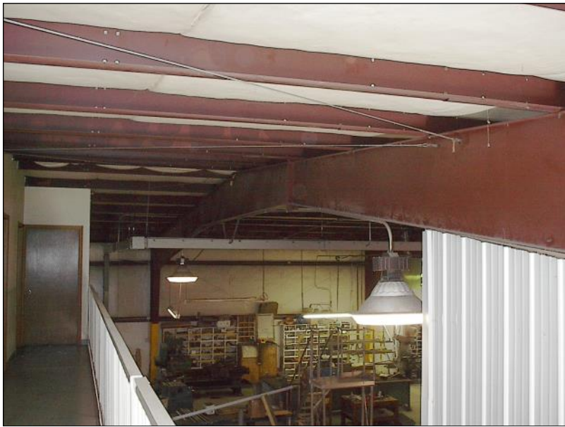
Side Ceiling View 72 ft Clear Span Red Iron.
